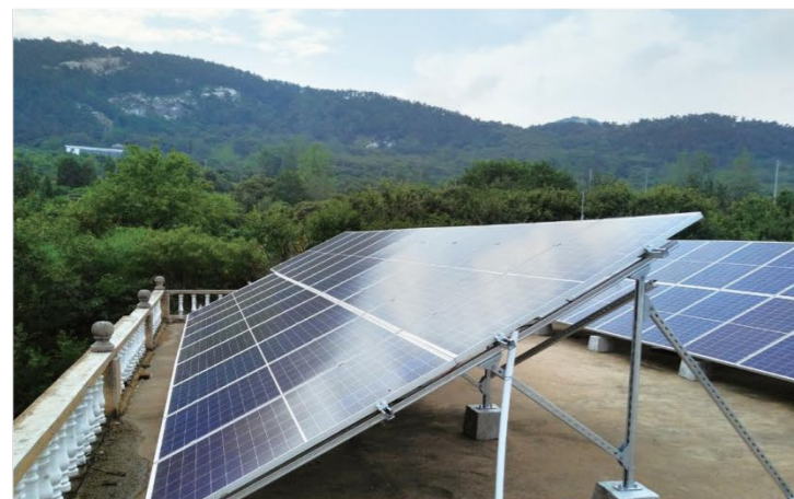
Grinding Project Shantian, Linshu County, Linyi City, Shandong Province
